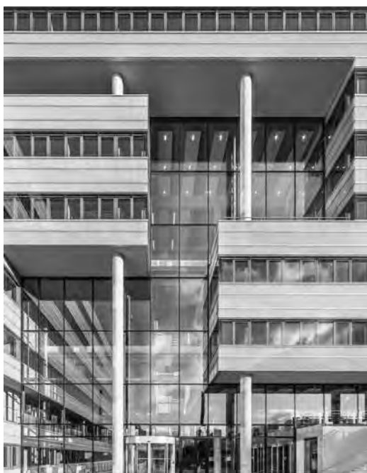
6. Herman Hertzberger, Laurens Jan ten Kate, Harm Freymuth, Maartje Nuy, Paul van Dijk, Oscar Backus, Faculty of Applied Physics and Electrical Engineering, Flux, Eindhoven University of Technology, Eindhoven, 2014. Dettaglio del fronte d'ingresso a ovest. Foto Norbert van Onna. Courtesy AHH.
